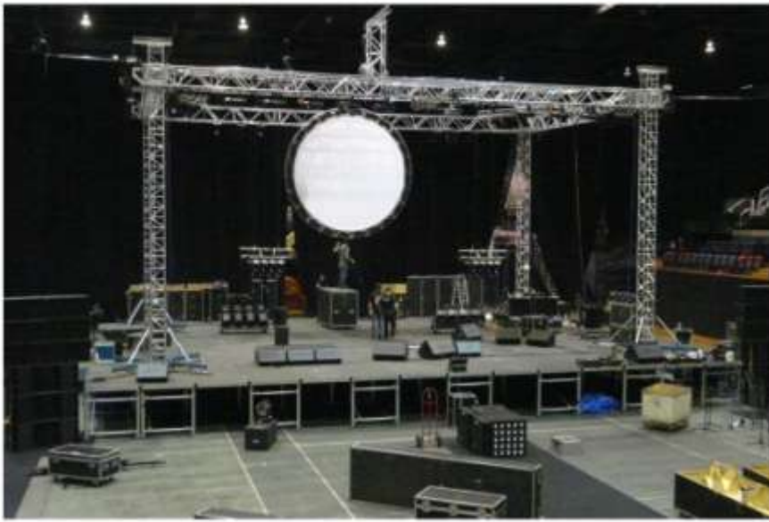
Above: A Typical truss system set up
